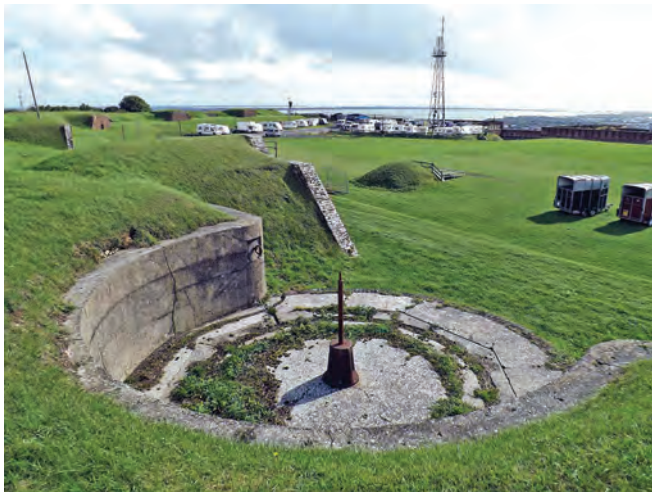
A gun pit for a 68 pounder RML on the ramparts at Fort Widley; the gun would have faced inland. Note the parade ground in the background. The mound behind the emplacement is the top of the spiral staircase down to the main magazine (later emergency centre) and caponiers
